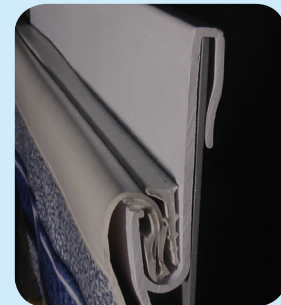
If bead receiver is too large, just peel off vinyl wedge lock and insert behind liner bead to secure bead
